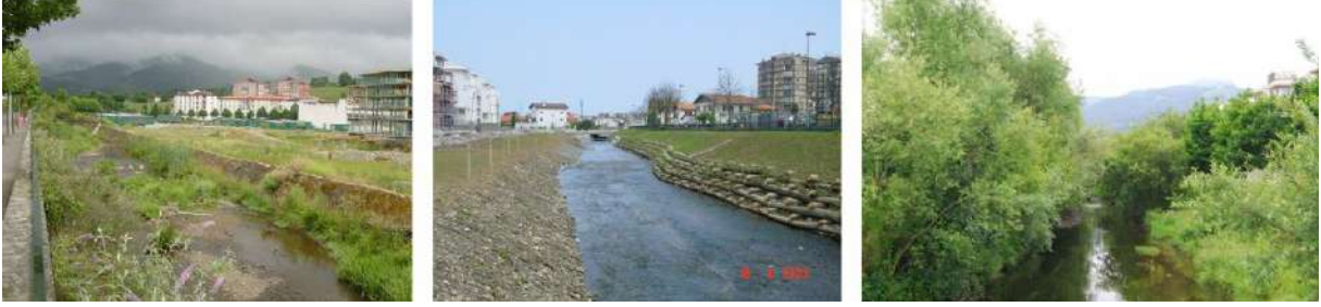
Restauration of the Artia Channel with Soil and Water Bioengineering
